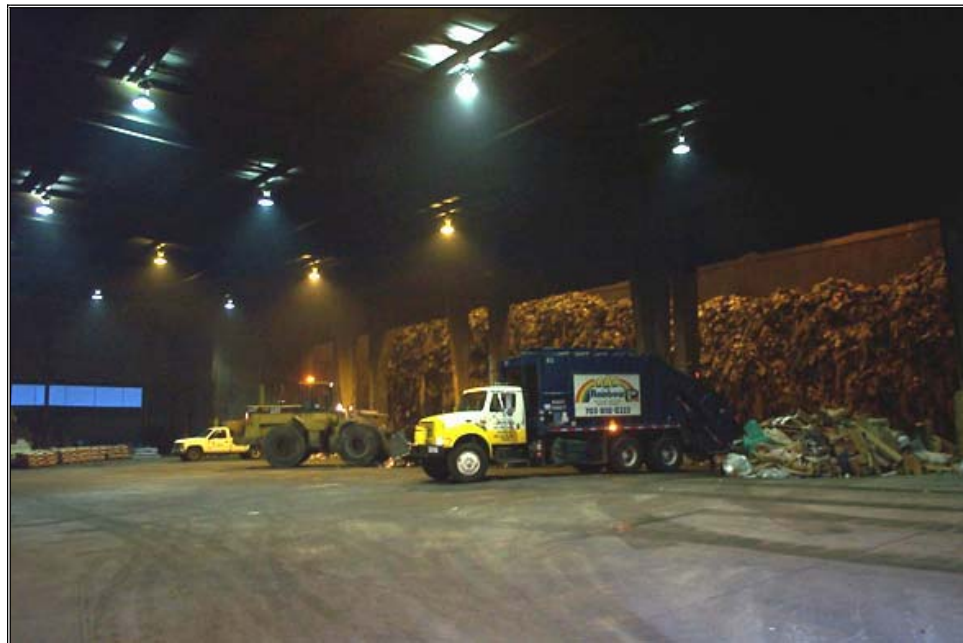
Alexandria/Arlington Tipping Floor
