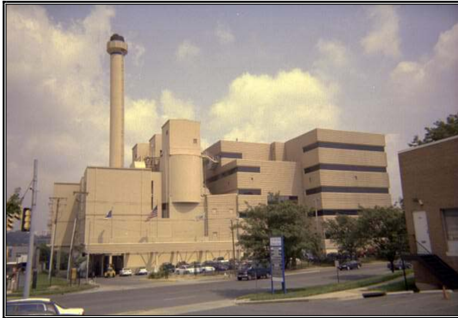
Alexandria/Arlington Waste-to-Energy Facility
