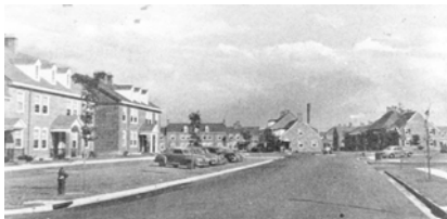
It takes a lot of work to maintain an historical community like Fairlington Commons.
